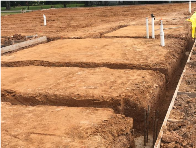
3. Excavation of grade beams
