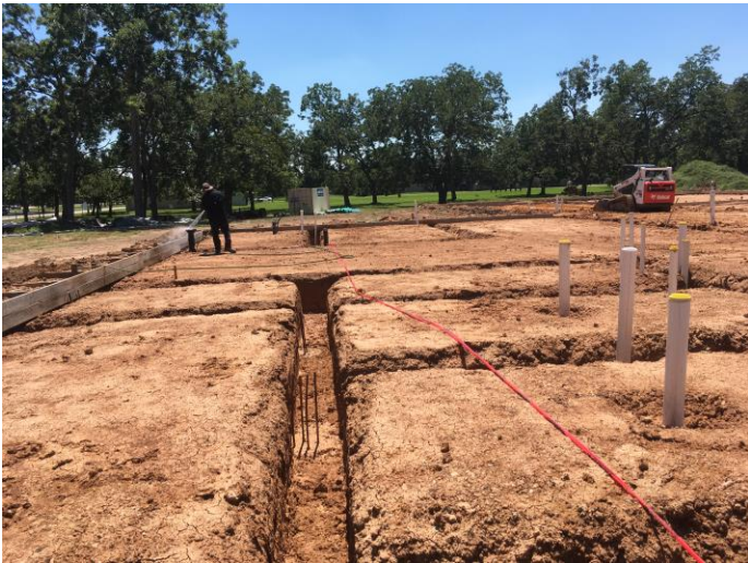
1. Pretreat of subgrade for termites
