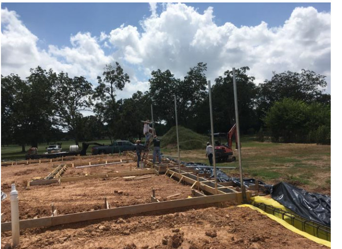
6. Installation of fence post at large animal area
