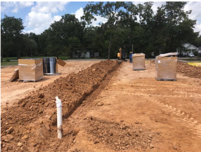
5. Trench drain subgrade excavation
