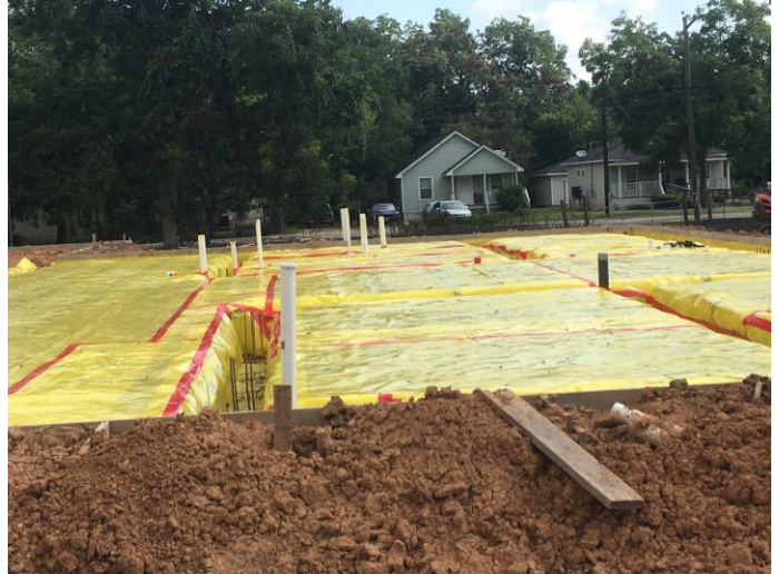
2. Installation of vapor barrier
