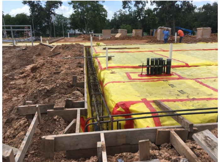
4. Grade beam reinforcing steel placement
